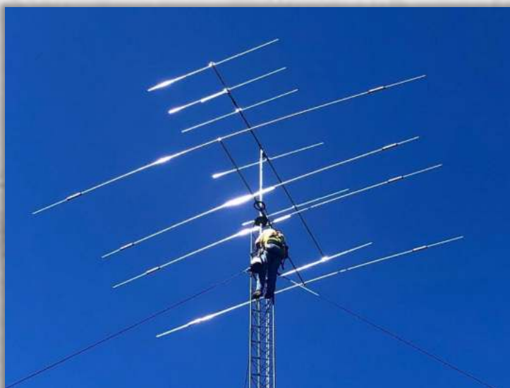
Adam Blackmer, K7EDX, does final installation of a Mosley TA-33MW (below a 6m Yagi) in September 2020 at W7UUU
